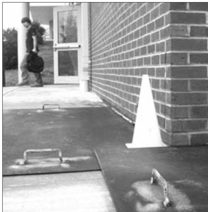
Specially fabricated steel lids cover the spots where Rocket Arena was core drilled and tested.
