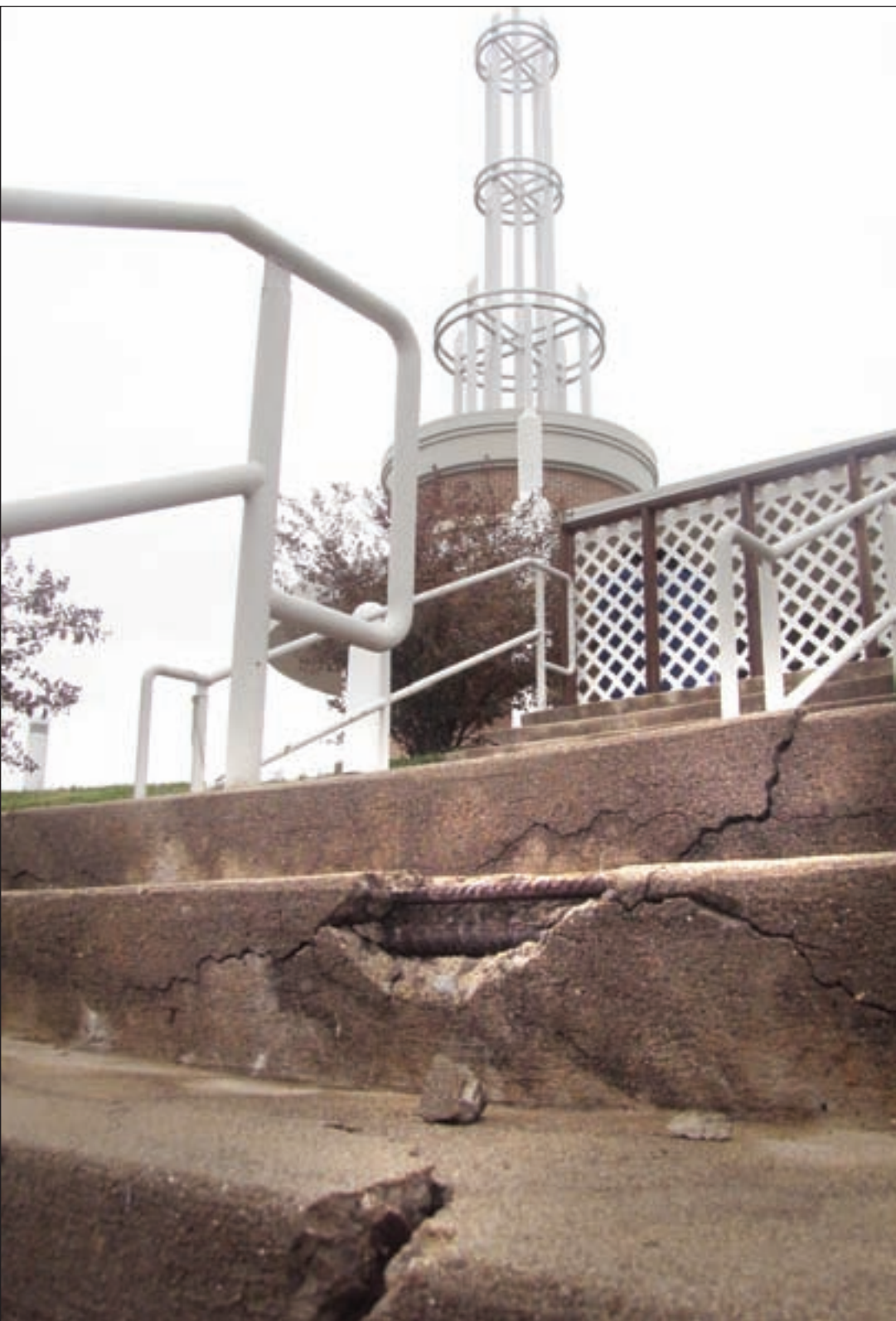
Concrete steps leading to Rocket Arena have been deteriorating and blocked off from public use for more than two years while the matter was being settled in court. School officials say the flatwork – steps and sidewalks – should be replaced in the spring.
